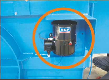
Automatic central lubrication system for the screw bearing (series)
